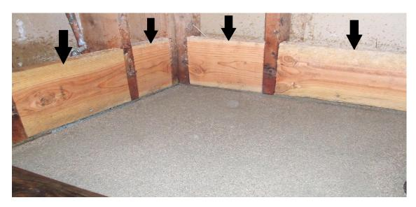
• Curbs also commonly called the Dam are most commonly constructed of three 2X4¢s stacked oflato on top of each other. What determines the height of the Dam is where the odrain topo height is. The Dam should be a minimum 20 higher than the top of the drain. Put a level on top of the drain and make sure the Dam is higher to hold water from leaking over.
